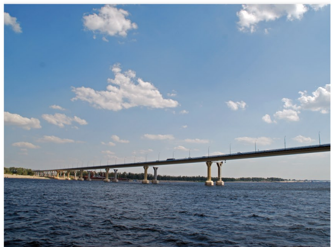
Photos courtesy of Cavin (@flickr.com) - granted under creative commons licence - attribution
